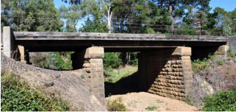
Figure 1 Bridge 62 near Kilmore East, Victoria
