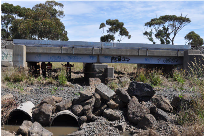
Figure 2 Bridge 44 near Little River, Victoria
