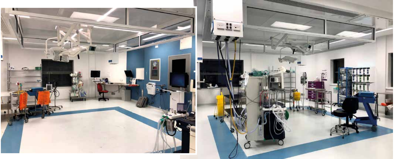
A modern UCV theatre. Note the demarcation to the floorcovering to indicate the canopy boundary. Even in modern UCV theatres, some of the largest of their kind, overcrowding from equipment can be a challenge, and should be considered when conducting performance tests and troubleshooting.
